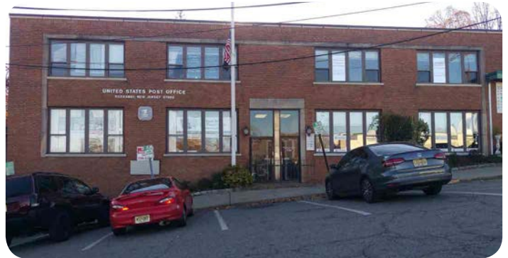
Rockaway Borough Post Office
